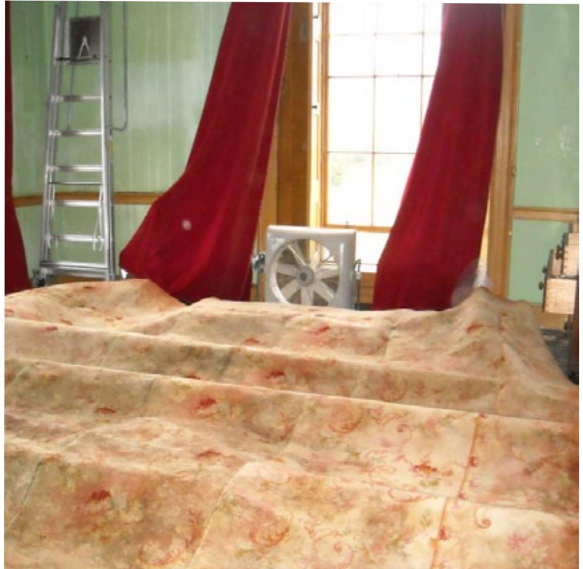
Above **The Study**: Underfelt removed, cold fans installed and the carpets propped on crates and pipes
